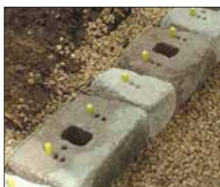
3. Insert Fiberglass Pins
