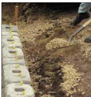
4. Install Fill & Compaction
